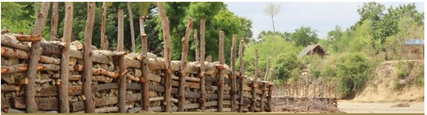
Dyke construction under WFP cash-for-assets project in Pauk Township, Magway ©WFP
